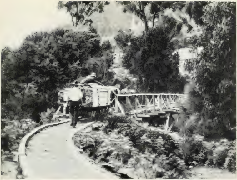
FIG. 71. FOREST TRAMLINE WITH WOOD RAILS : AUSTRALIA. [By courtesy of Government of Victoria.]
